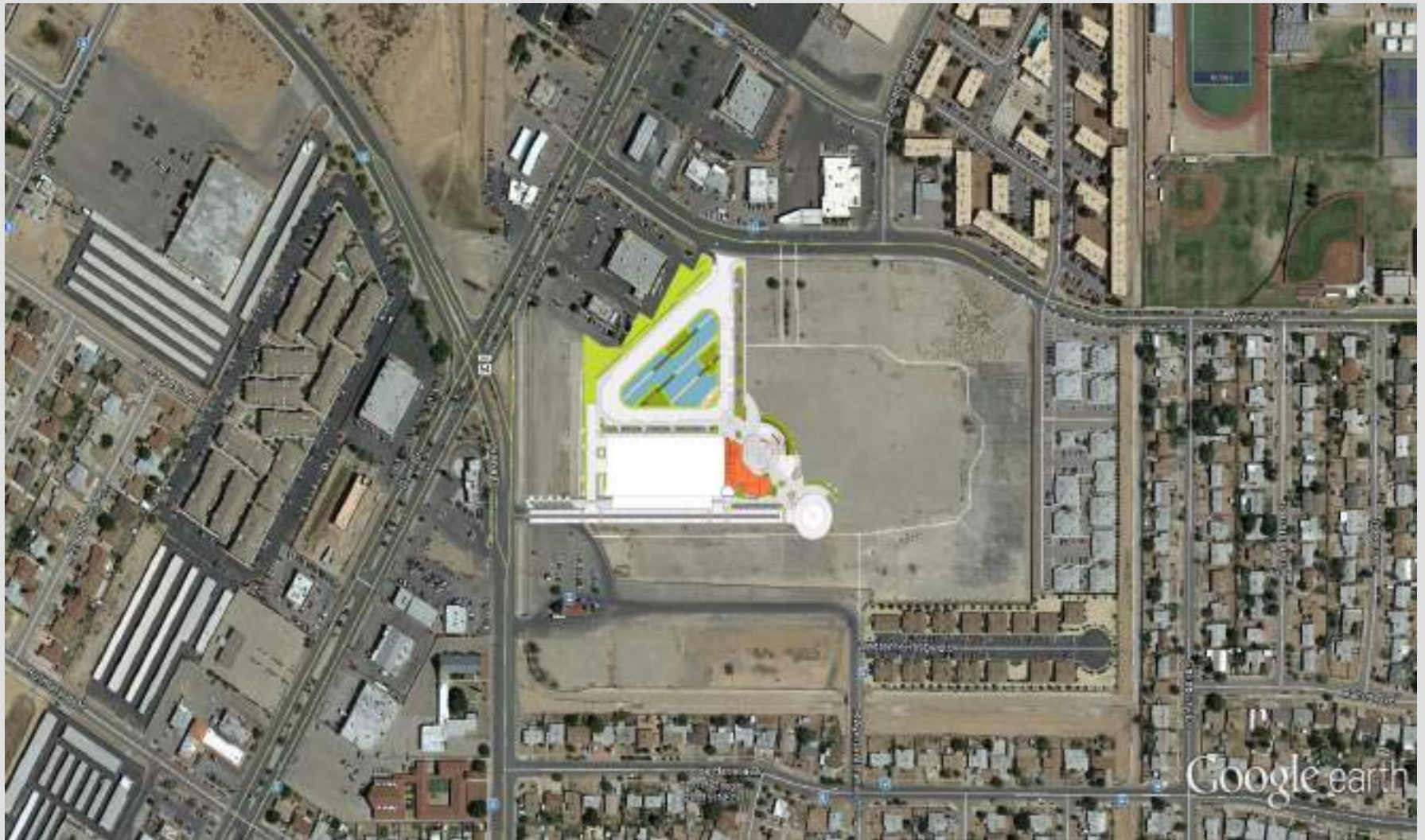
Aerial View of Northeast Property (After)
